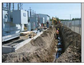
Construction underway at the substation in Fort Albany for the connection of the spare transformer.
